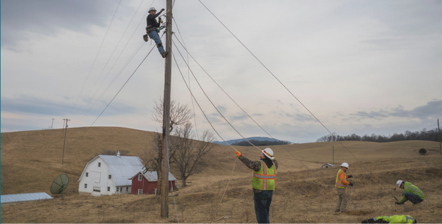
Workers install fiber optic cable to expand broadband coverage.
